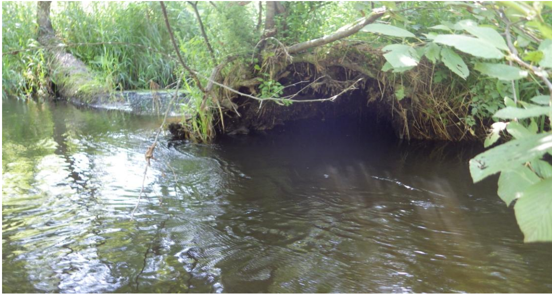
Figure 9: Photos of Some of the Severe Erosion in the Watershed
