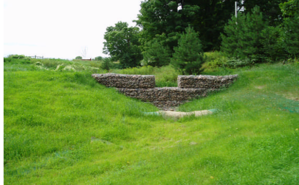
Rock Gabion in restored Swale
