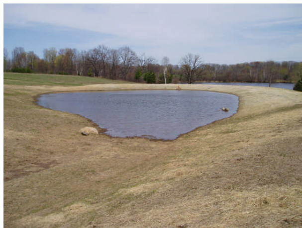
Olson Pond at Beginning of Restoration
