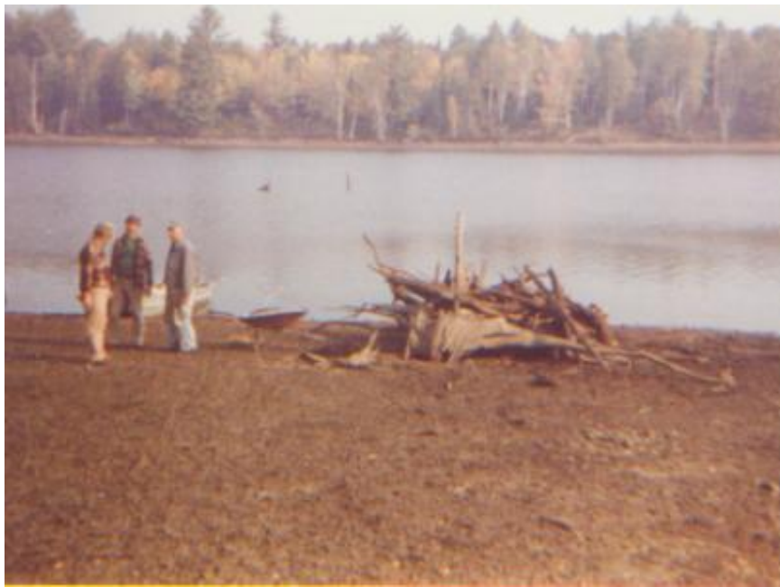
Building a fish crib during the draw down on Lake Alice -- September 1983.
