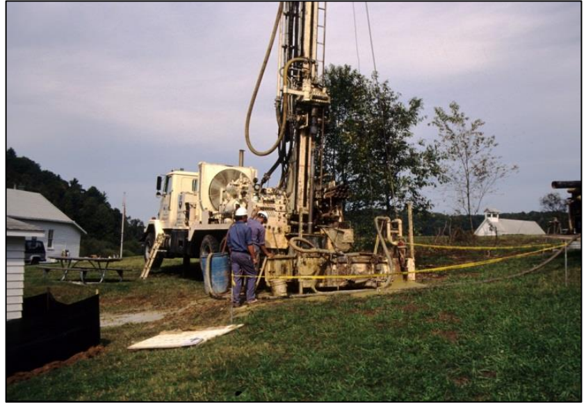
Drilling a well on rural property.
