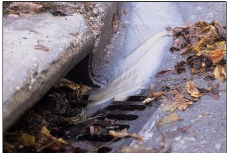
Storm water drain receiving runoff.
