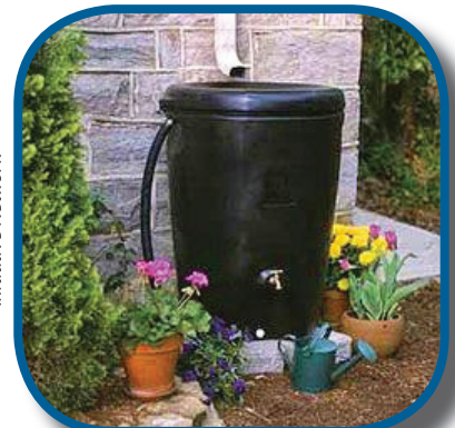
Green roofs, left, and rain barrels, above, catch stormwater runoff.
