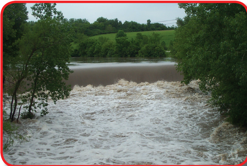
The Horlick dam must be upgraded to safely pass floodwaters.
