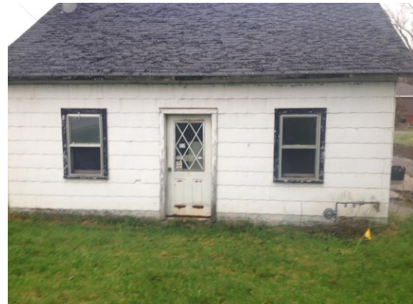
Former shop, west side
