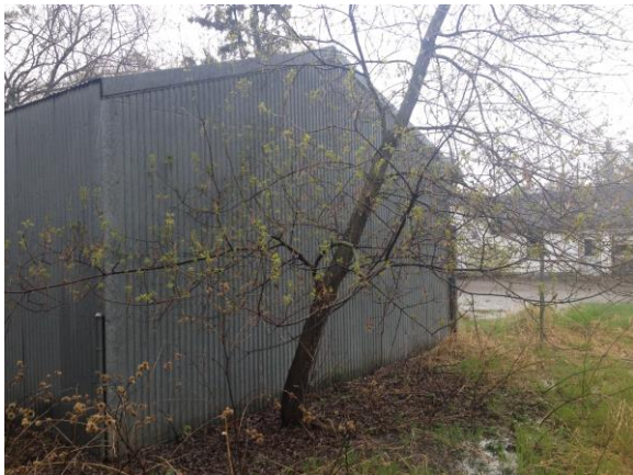
Garage, east side
