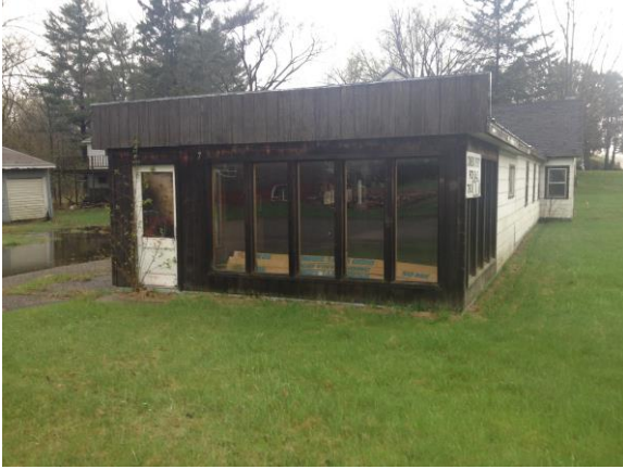
Former shop, east side
