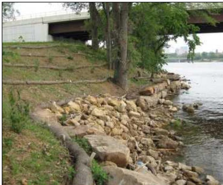
**Figure 26. Riprap here was placed carefully from the bottom of the slope to preserve the existing trees. This may be possible at some sites where access is permits**
