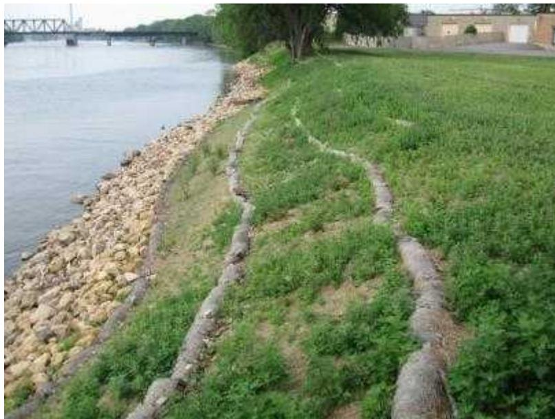
**Figure 28: Water levels move up and down frequently at this site, keeping vegetation from developing among the riprap.**
