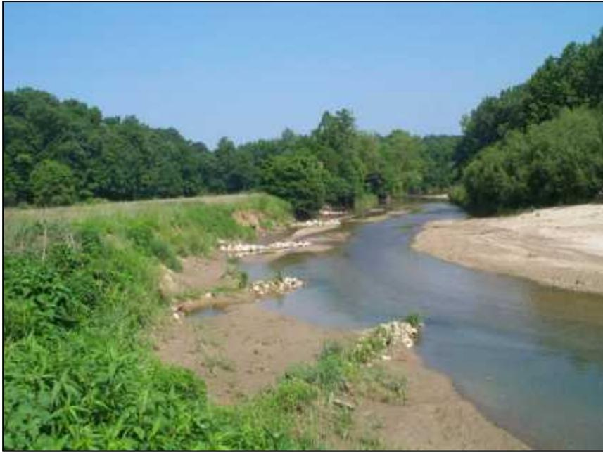
**Figure 29: Rock/riprap barbs forcing the flow to the right and catching sand on their downstream sides.**
