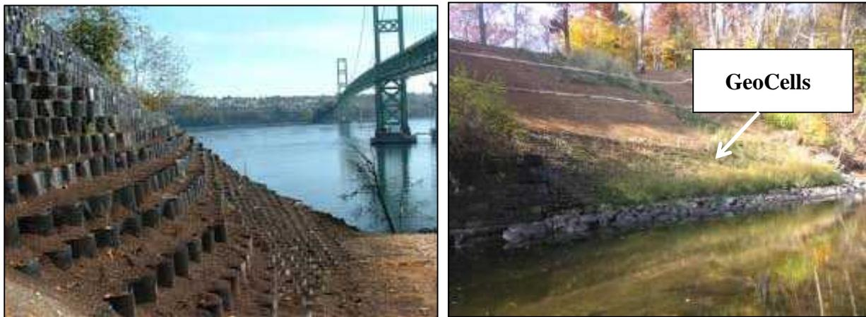
**Figure 34. Example of geocells being used along steep banks. The cells are filled with soil and then vegetated. They are usually used in concert with riprap or wood along the bank toe.**
