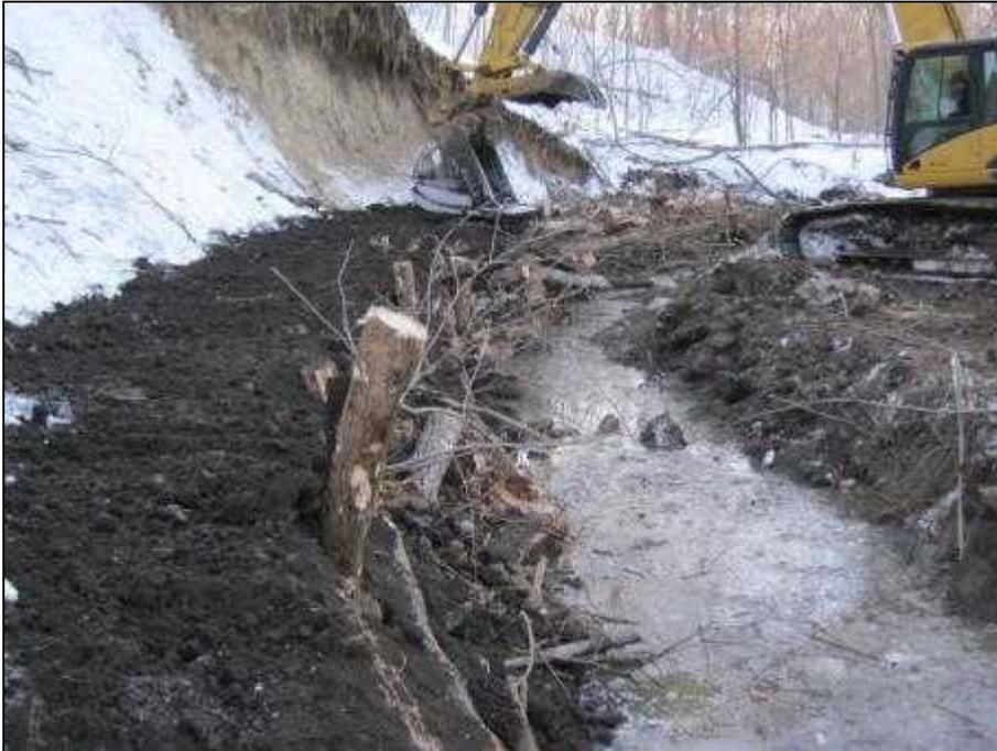
**Figure 32. Example of a large wood cribwall under construction at the toe of a failing sand bluff in Minnesota. The space between the interlocking logs was filled by additional wood and rock, before being covered with soil. After construction, the bench will be planted with native vegetation.**
