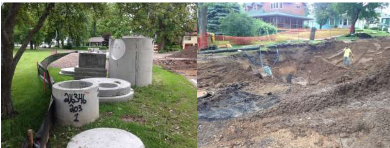
Figure 15 – Humbird Street Grit Chamber Installation
