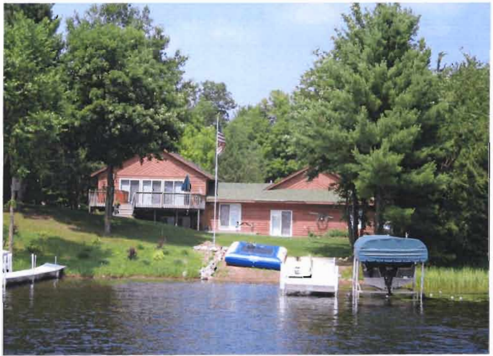
Figure 12. Both of the pictures are from Pipe Lake. [top] This parcel would rate as having a shoreline with a buffer greater than 50% of the lot width and an understory (ground cover) with greater than 50% natural cover. [bottom] This parcel would not qualify as having a natural shoreline buffer greater than 50% of the lot width. Also the understory in the upland area is dominated by lawn cover and would be rated as having less than 50% natural cover.
