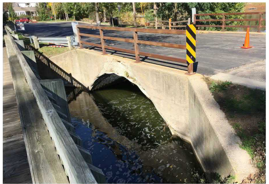
Figure 1.1 Ferry Drive Existing Culvert
