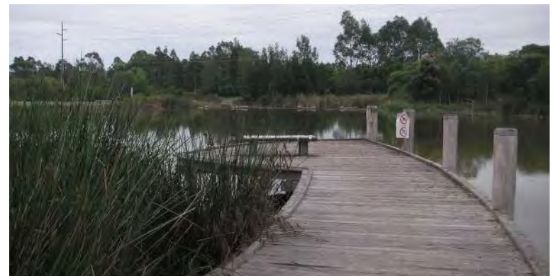
Opportunity to Provide ADA Accessibility
