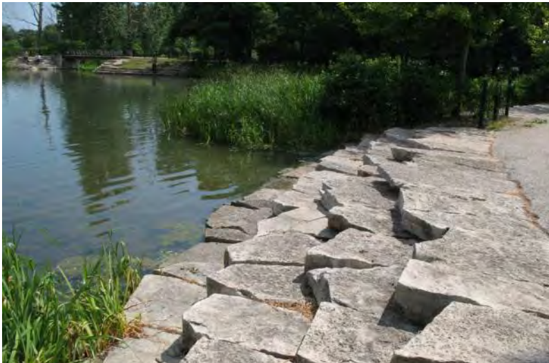
Stone Steps Accommodate Fluctuating Lake Depth
