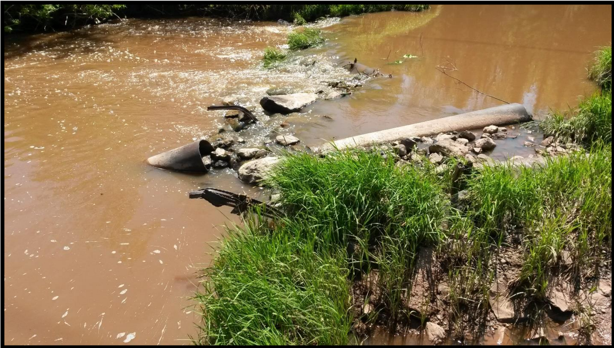
Figure 13. Remnants of old concrete sewer lines are sitting in the Pokegama River
