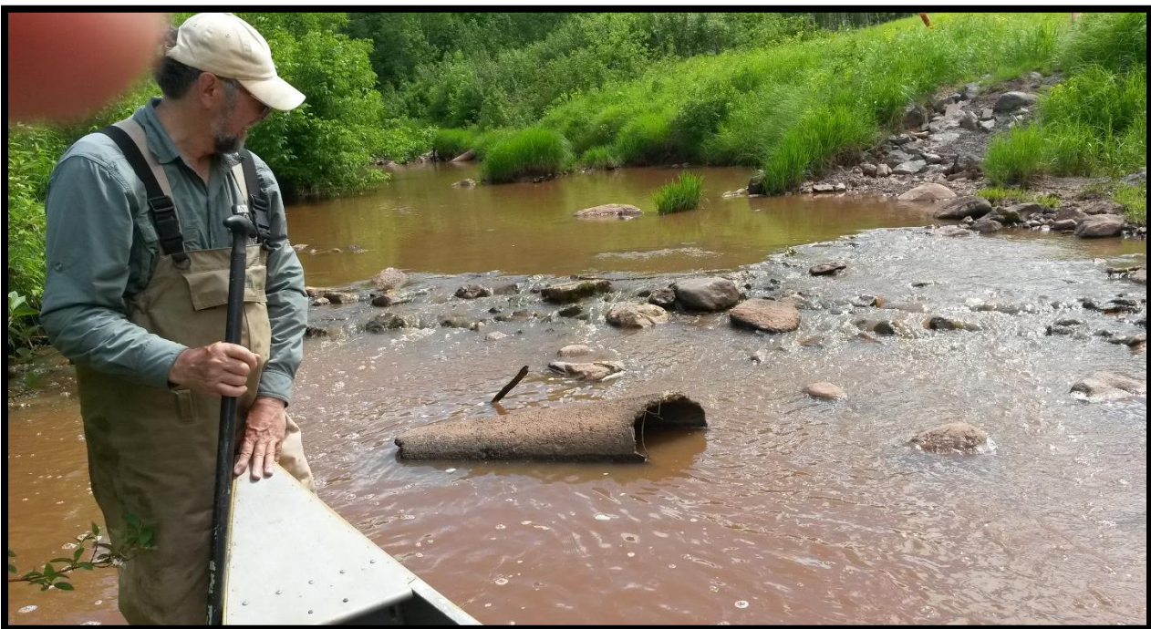
Figure 13. Remnants of old concrete sewer lines are sitting in the Pokegama River
