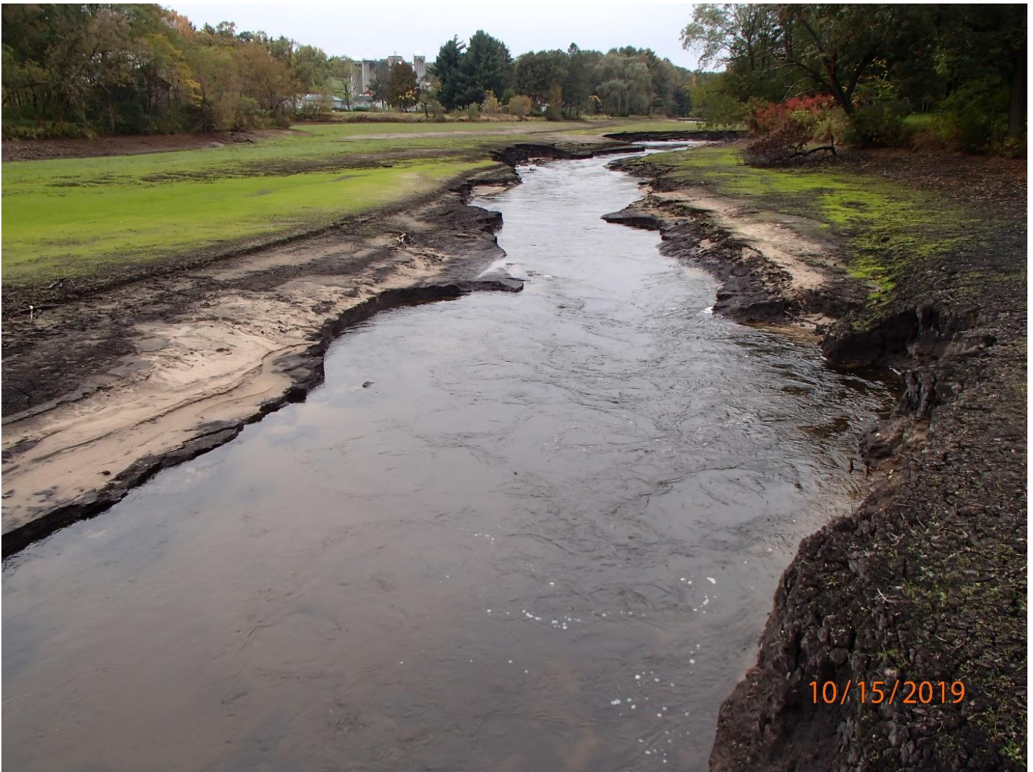
Photo 5: Drawdown of the Pine River Millpond in 2019 for Spillway Maintenance. Photo taken by D. Bolha on October 15 th , 2019.
