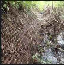
UNTtoGarnersCk@cThKK-Noe b ad restoration (4)
