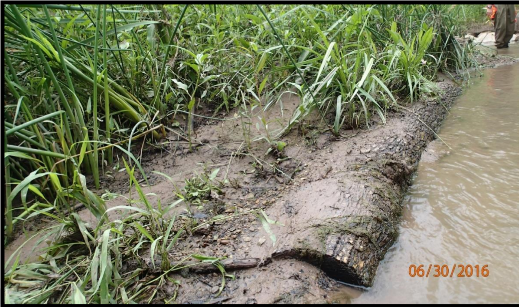
Log Vanes for sediment sequestration and bank stabilization
