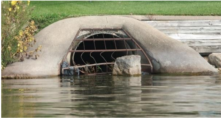
Point Source – look for a pipe bringing water directly to the lake. This pipe could be directing stormwater, gray water, or other water sources to the lake.
