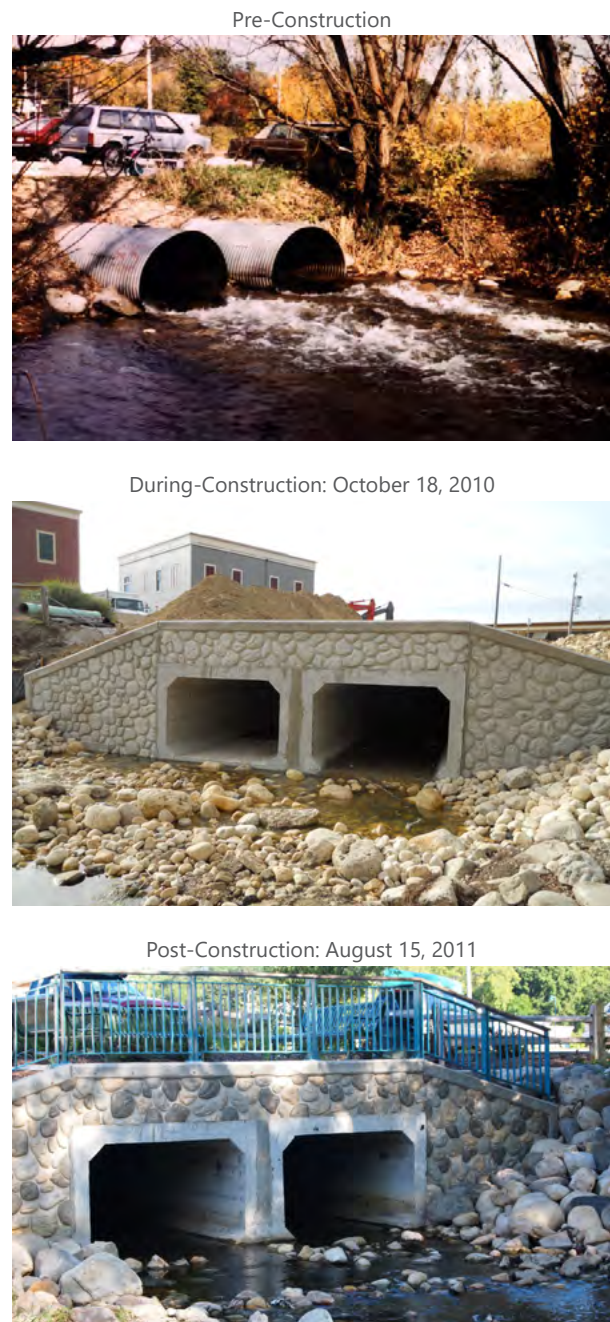
Figure 2.20 Pewaukee Lake Dam Outlet Infrastructure Configuration
