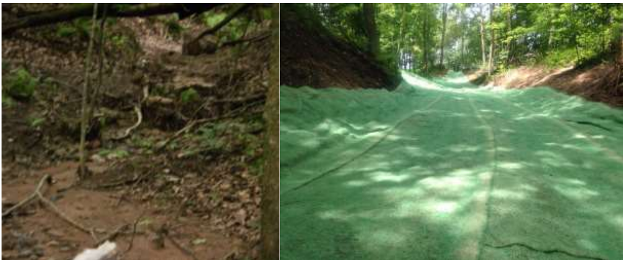
Figure 16: NW Wash repair project (LEAPS, 2016)
