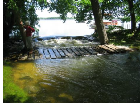
Water pours through the Lake Ripley outlet and floods the adjoining property following a 2008 high-water event.
