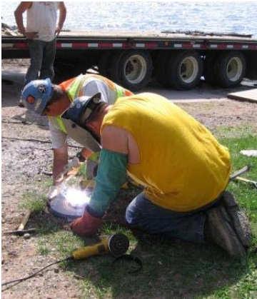
Welding Footing Plate on Pier
