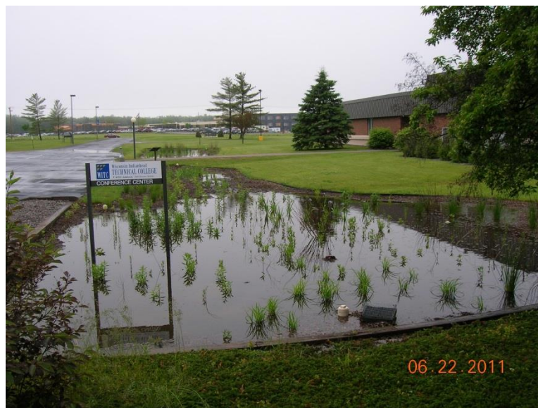
Figure 20. A newly-installed rain garden in Ashland stores runoff after a heavy rain event.
