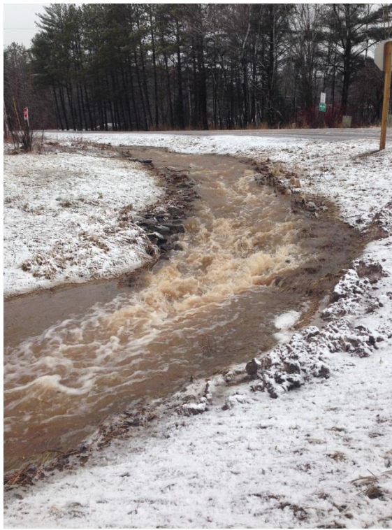
Figure 21. Roadside ditch during spring thaw carrying sediment-laden runoff to a stream or lake. Photo courtesy of Michele Wheeler.
