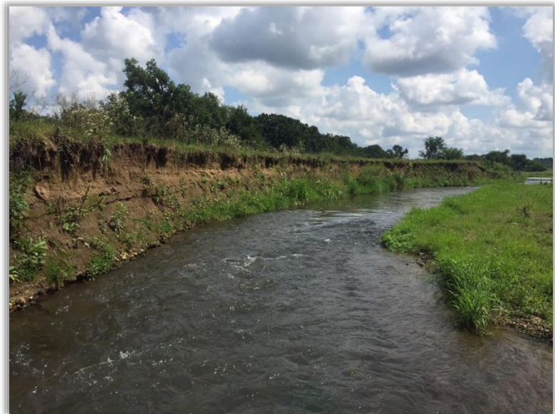
Sinisawa River upstream of Sinisawa Road. Streambank erosion on the left bank.
