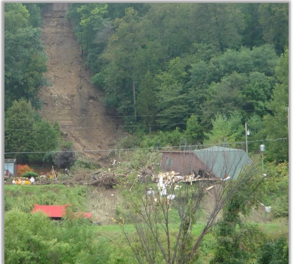
Mudslide to Mississippi River and consequent property loss. Fifteen inches of rainfall over a 24-hour period triggered the slide.
