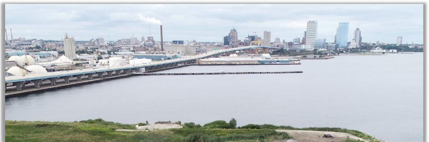
Location of the new Dredged Material Management Facility in the Milwaukee Estuary Area of Concern. Photo credit: Milwaukee Metropolitan Sewerage District.
