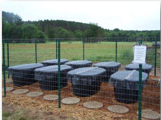
Temporary fencing and informational signage will tell curious bystanders that the tanks are part of your special lake-improvement project.
