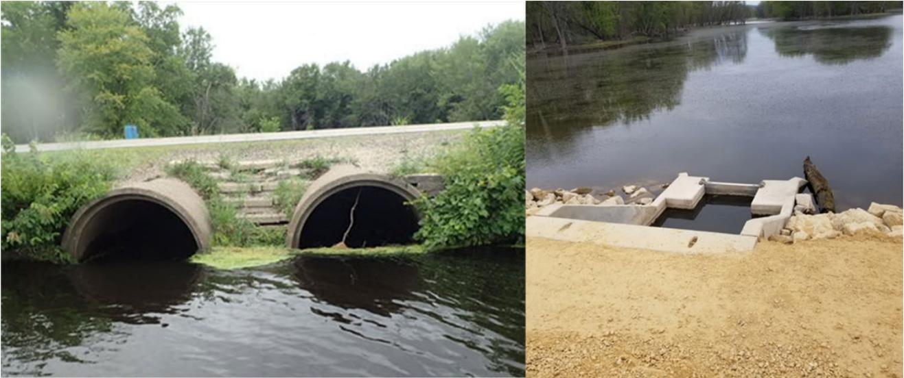
*Figure 22: Photo on left shows uncontrolled culverts. Photo on right shows the climate adaptation design with water control via stoplogs up to river elevation of 632 feet. At water surface elevation greater than 632 feet, water is uncontrolled.*
