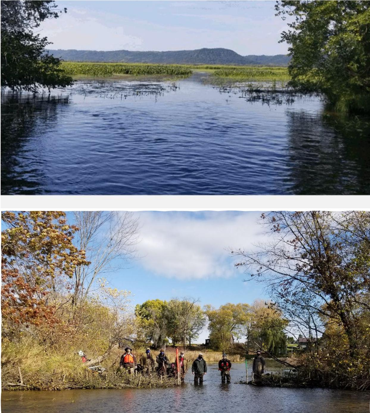
*Figure 26: Top panel: Levee breach prior to buckthorn bundling project. Bottom panel: Post-project breach reduction using the buckthorn brush bundling technique.*
