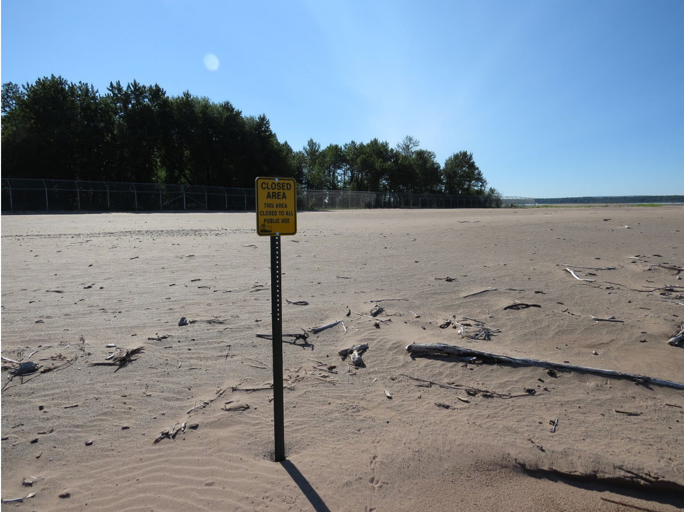
Completed site and fence (2020)
