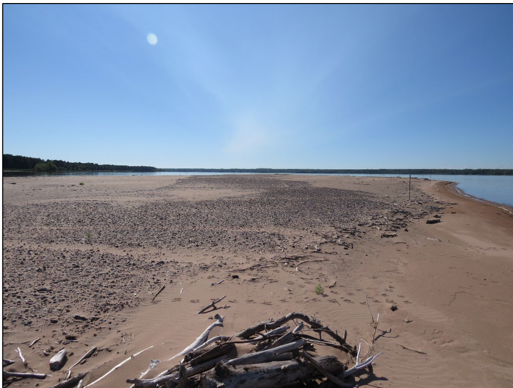
completed cobble pan
