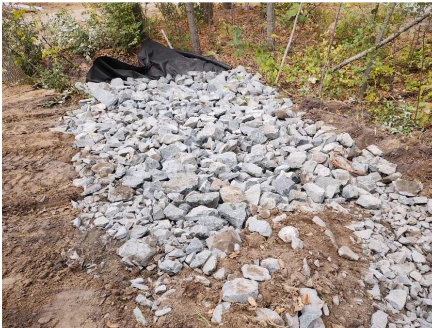
Date Pictures taken: 10/24/2020 Description: Rock infiltration pit installation
