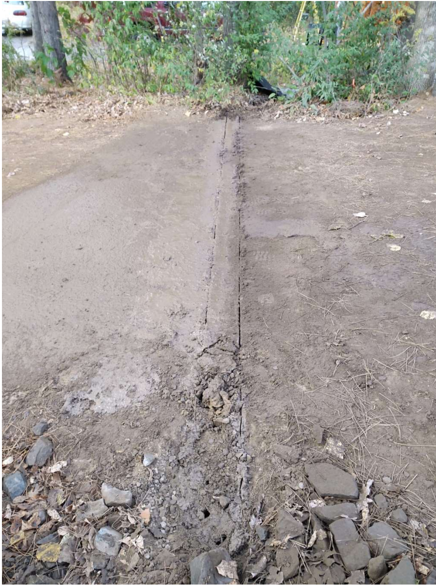
Date Picture taken: 10/24/2020 Description: Diversion trench cut out
