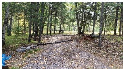
Photo 27: Sep 21, 2020. Two conveyor belt diversions with rock outlets installed.
