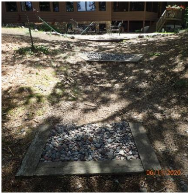
Photo 22: Top 2 infiltration pits.
