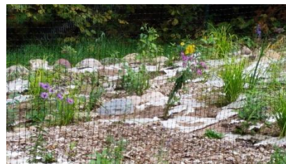
Photo 41: Sep 21, 2020. Native plants were used. Terracing was used to help slow down water on the slope.
