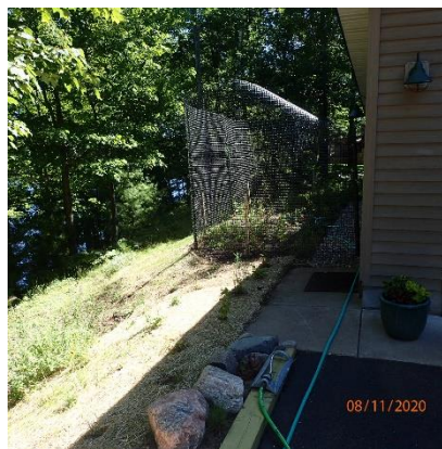
Photo 35: Aug 11, 2020. Rain garden area is contained on flat area before slope.
