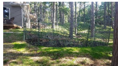
Photo 6: Sep 3, 2020. Rain garden installed.
