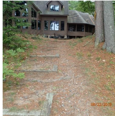
Photo 16: Aug 22, 2019. The access path had timber framed steps.
