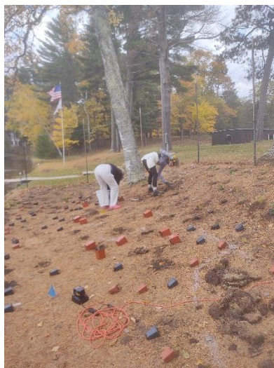
Photo 10: Oct 6, 2020. The volunteers started installing the plants.
