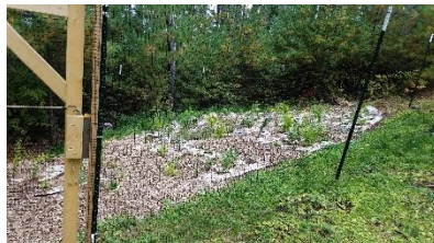
Photo 40: Sep 21, 2020. A rain garden and deer fencing were installed to manage stormwater from the dorm.
