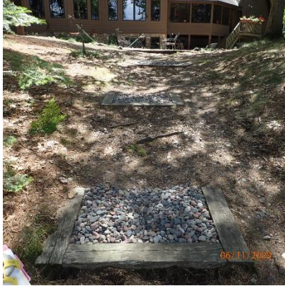
Photo 21: June 11, 2020. Three infiltration pits are installed.
