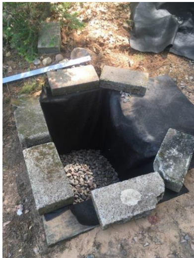
Photo 19: June 9, 2020. Pit is lined with filter fabric on all sides and filled with rock.
