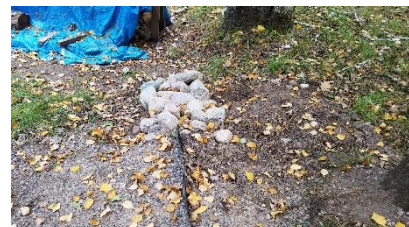
Photo 29: Sep 21, 2020. Rock outlet at end of diversion.
