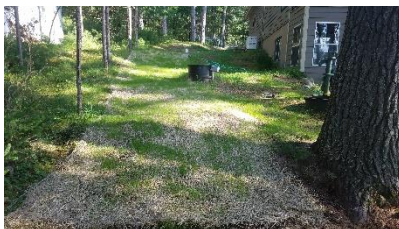
Photo 4: Sep 9, 2020. Two broad-based dips were installed and seeded along driveway.
