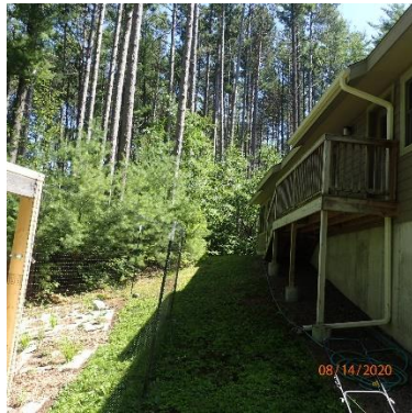
Photo 37: Aug 14, 2020. While this photo shows the rain garden on the right, it shows the roof runoff, gutter, and slope of the site.
