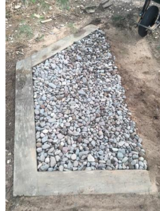
Photo 23: June 11, 2020. Top infiltration pit with 3 inches of rock over filter fabric.
