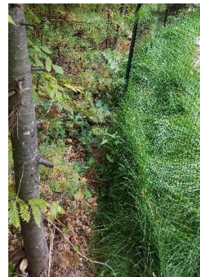
Photo 42: Sep 21, 2020. Even after several heavy rain events, the berm and outside area show no signs of runoff/erosion.
