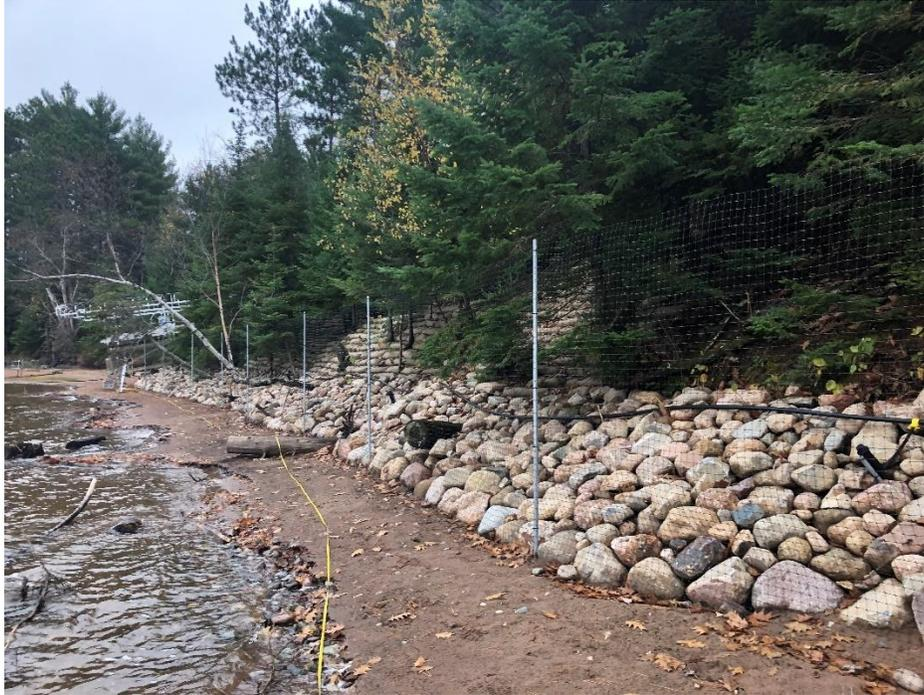
*Riprap protecting the toe of the bank and creating a stable foundation to build the vegetated geo-bag walls on. The riprap was installed to incorporate the existing trees that had fallen but were still rooted in the bank.*
