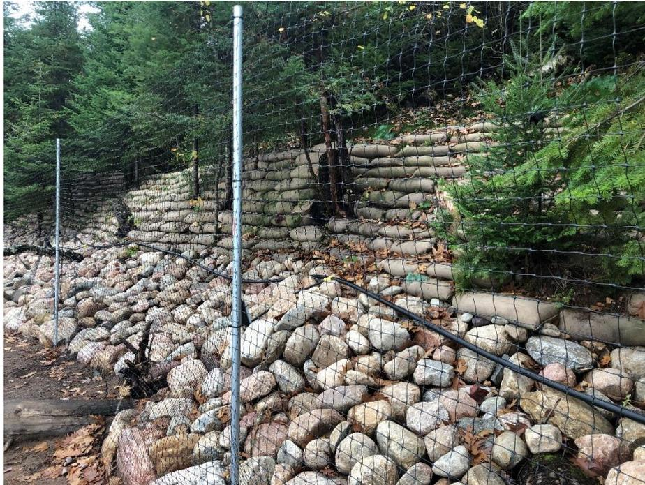
*Vegetated walls above the riprap incorporating the existing vegetation, each bag has two plants installed between each row. The black plastic pipe along the rock is the irrigation system and deer fencing was installed to protect the plants.*
