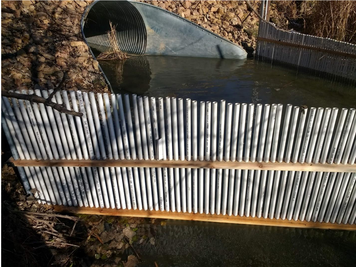
Figure 15. Lightweight carp barrier grate. (From Carp Solutions)
