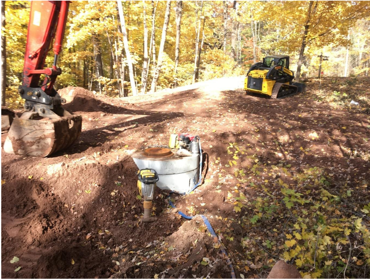
Photo 10. Final grading at Goldsmith site on Jeffery Boulevard
