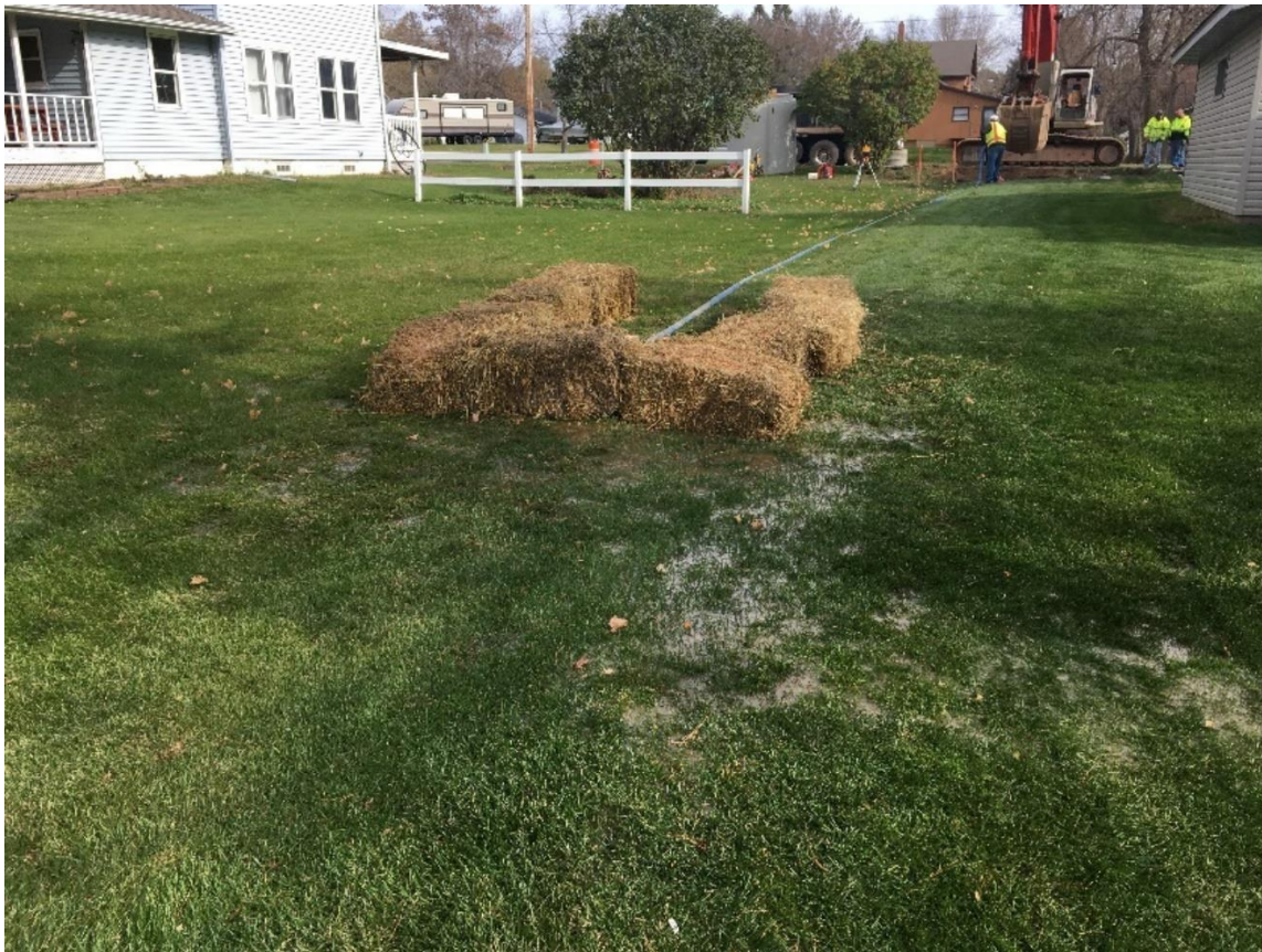
Photo 1. Dewatering at 3 rd Avenue project site during excavation
