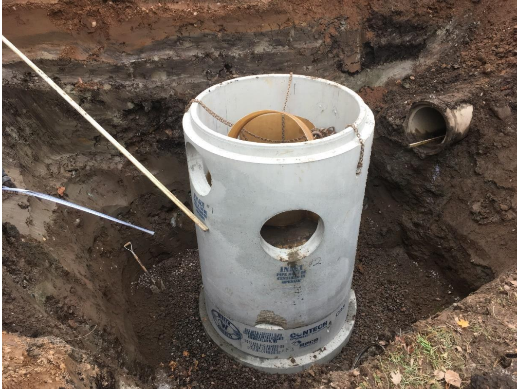
Photo 7. Installing hydrodynamic separator unit
