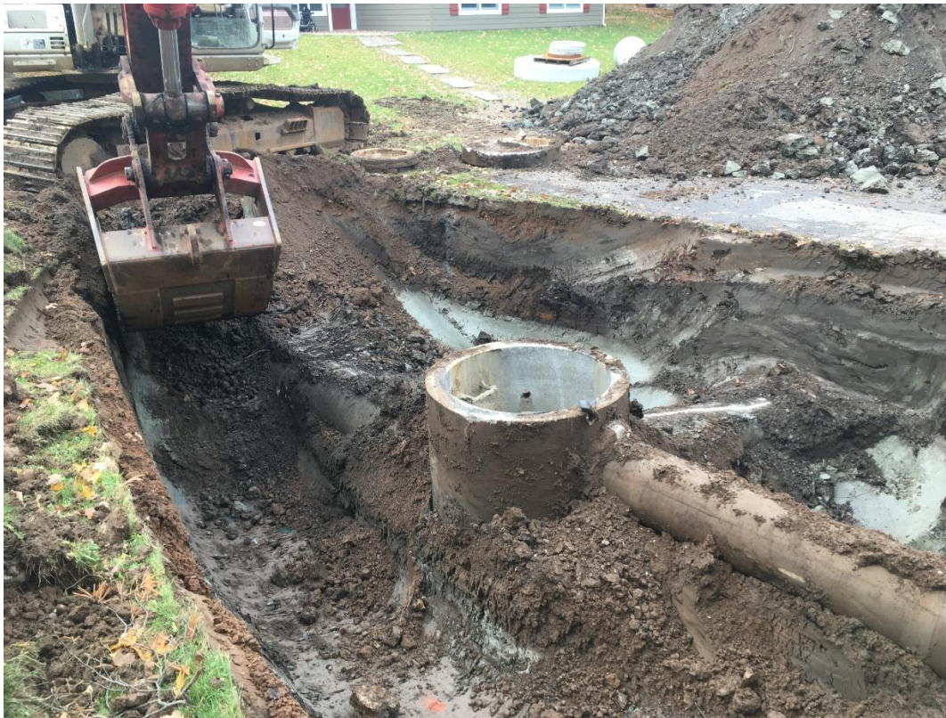
Photo 6. Excavation at Cifaldi site
