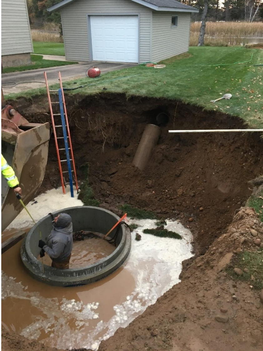
Photo 2. Installing hydrodynamic separator manhole at 3 rd Avenue
