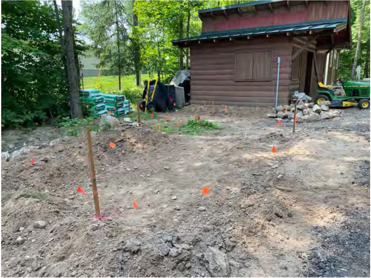
During construction pictures
