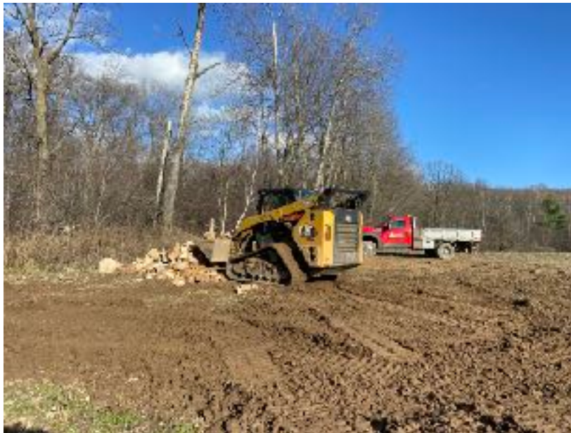
Landing area for equipment and materials
