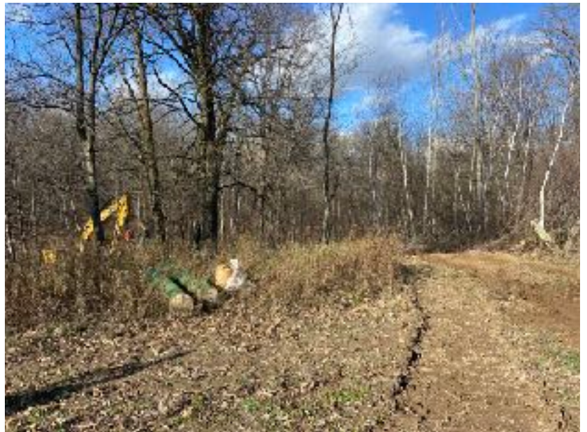
Site access from farm field
