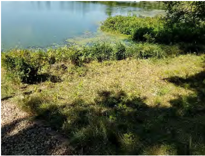
Photo 7: August 15, 2020 finished job
