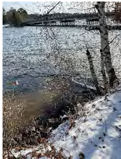
Photo 7: Winter of 2019 - 2020 finished job
