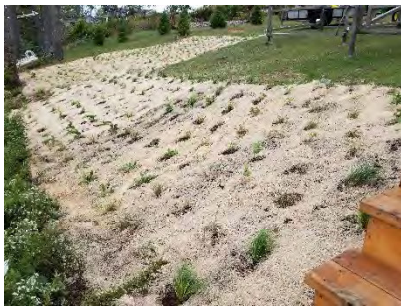
Photo 7: September 13, 2019 finished job
