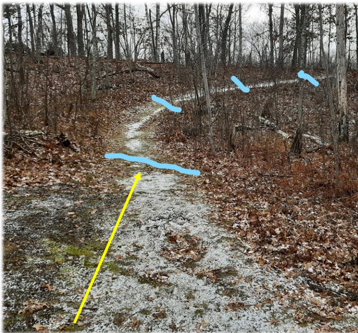
4 diversions installed along the path to lake
