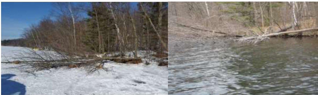
Figure 9: Fishsticks installation (left) and after ice out (right)
