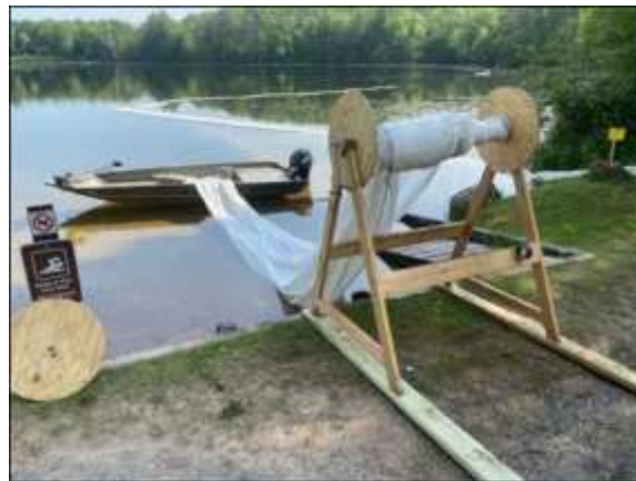
Figure 37: Limno-curtain material on a roll before installation (photo from Marinette Co. LWCD)
