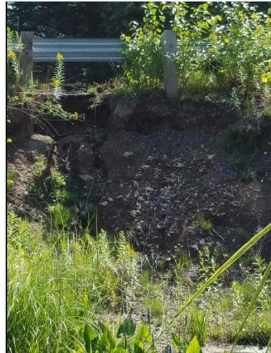
Figure 7. Erosion near Spring Creek Inlet crossing on Thousand Island Lake Rd.
