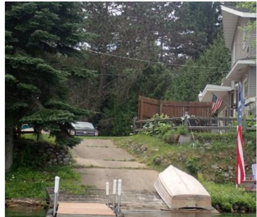
Figure 11. Impervious surfaces and straight trail access make a site even more prone to erosion. This site was augmented with a water infiltration pit to minimize runoff into the lake.
