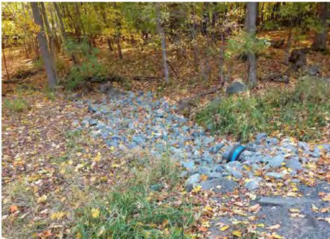
Before: 2, 4" culverts (partially blocked to be replaced by 1, 6" culvert, with pond elevation increased by 1.53 feet
