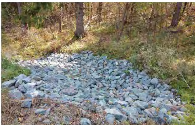
140 th Avenue Culverts – Johnson Preserve Outflow Stabilization, October 2020
