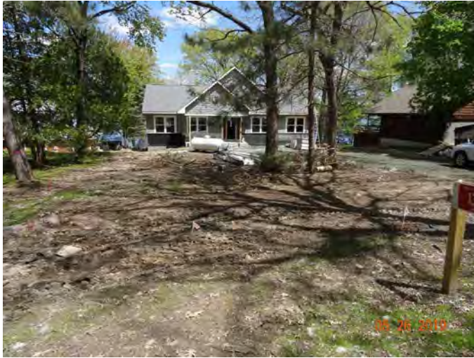
Before: May 2019 (Construction Site)
