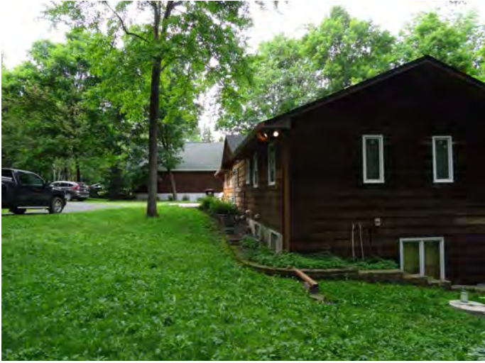
Before: Project will capture runoff from new garage (not shown) and parking area
