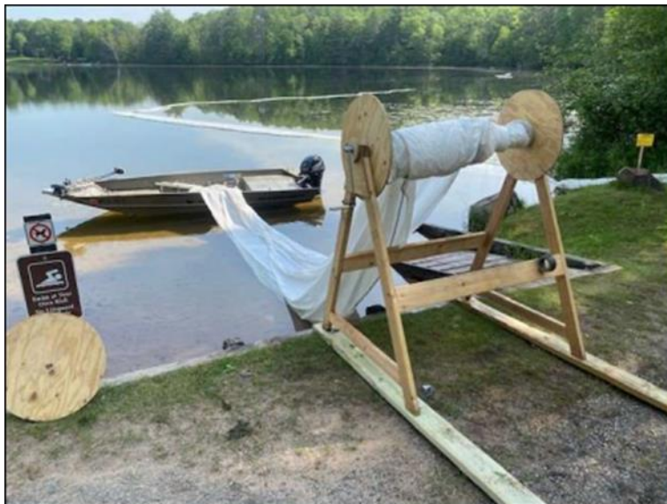
Figure 37: Limno-curtain material on a roll before installation (photo from Marinette Co. LWCD)
