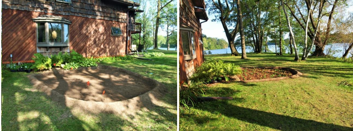
Figure 46: Rain garden installation (left) and upon completion (right)
