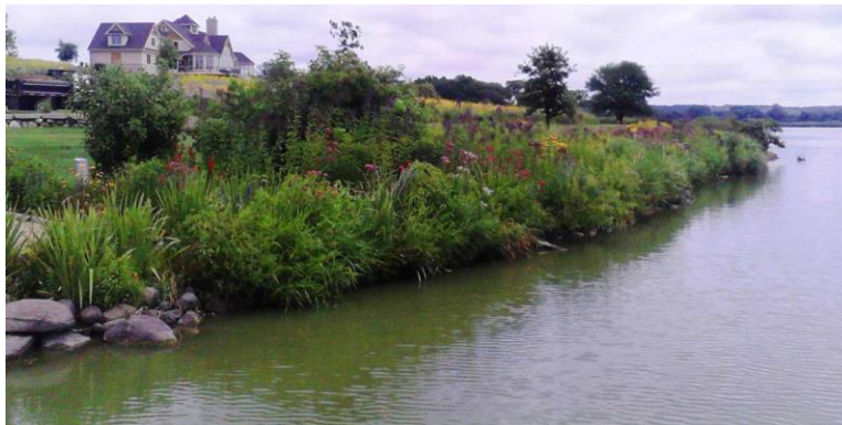
Figure 47: Completed native planting (photo from HealthyLakesWI.com)
