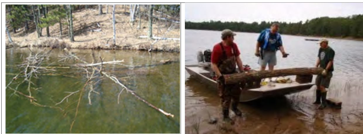
Photograph 8.6.6-3. Examples of fish sticks (left) and half-log habitat structures. (Photos by WDNR)
