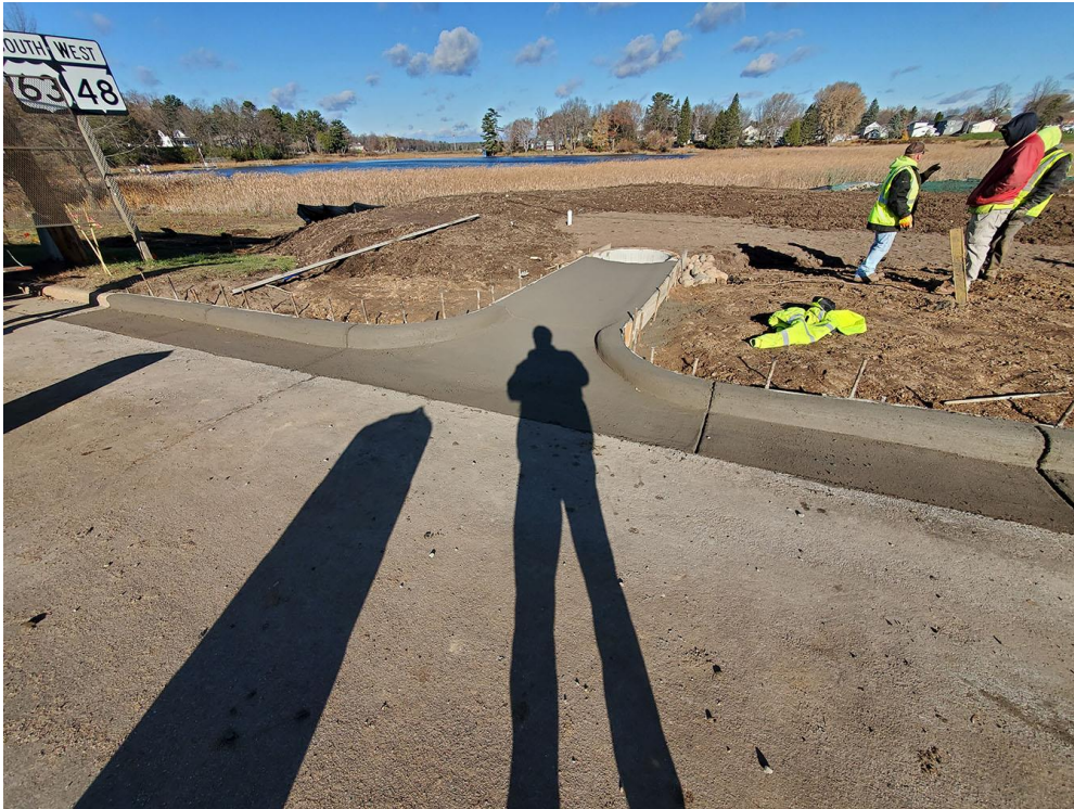
Figure 4. Rain garden inlet installation, November 9, 2023
