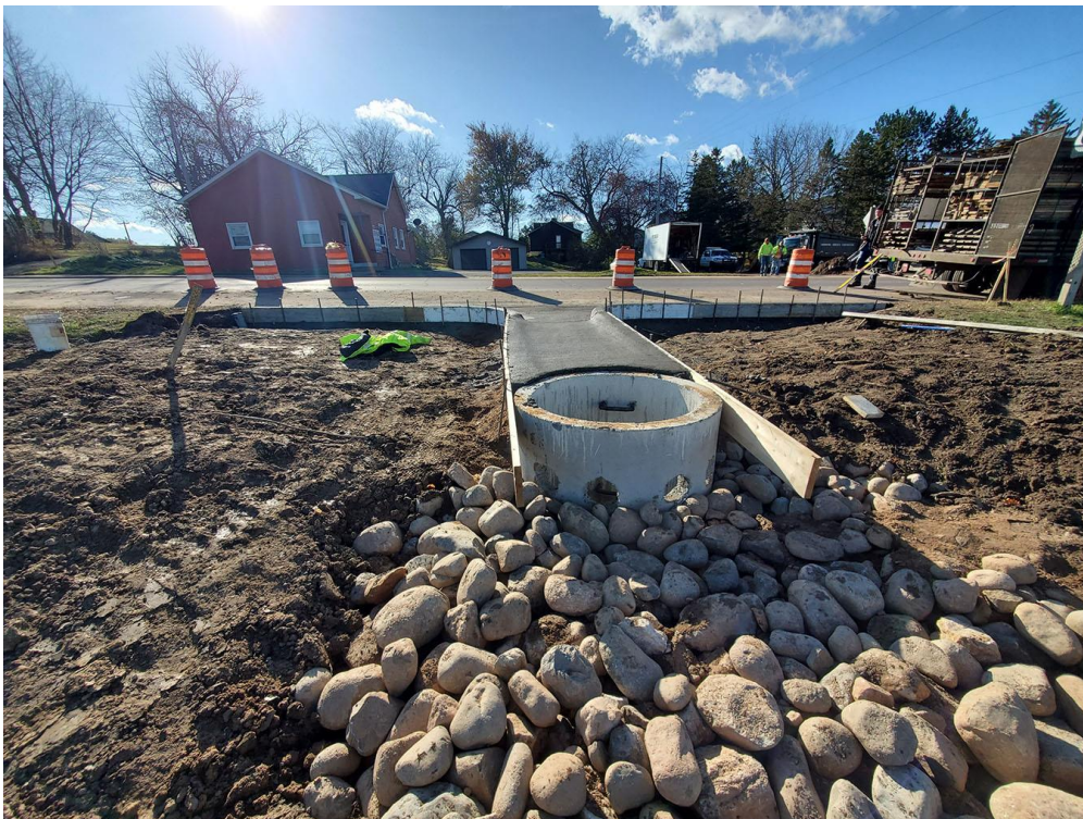
Figure 3. Rain garden inlet installation, November 9, 2023
