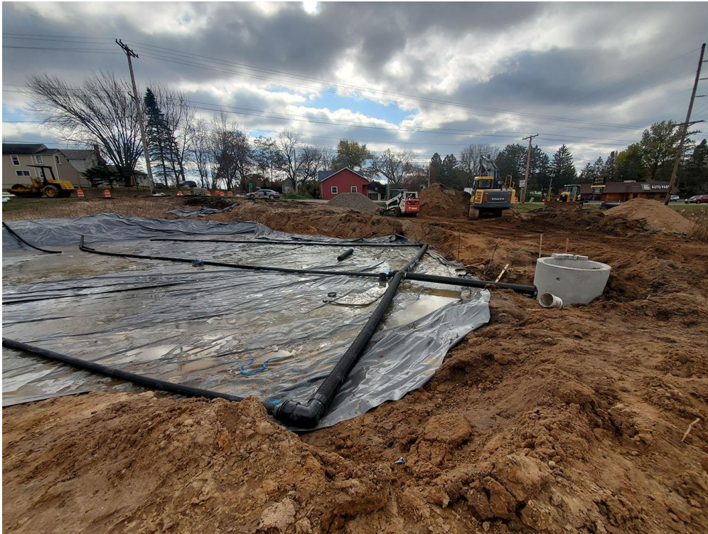
Figure 2. IESF drain tile installation, October 30, 2023
