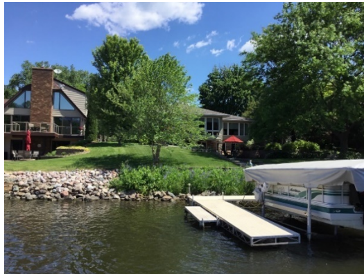
Shorelines: rip rap (left) and natural/restored (right).
