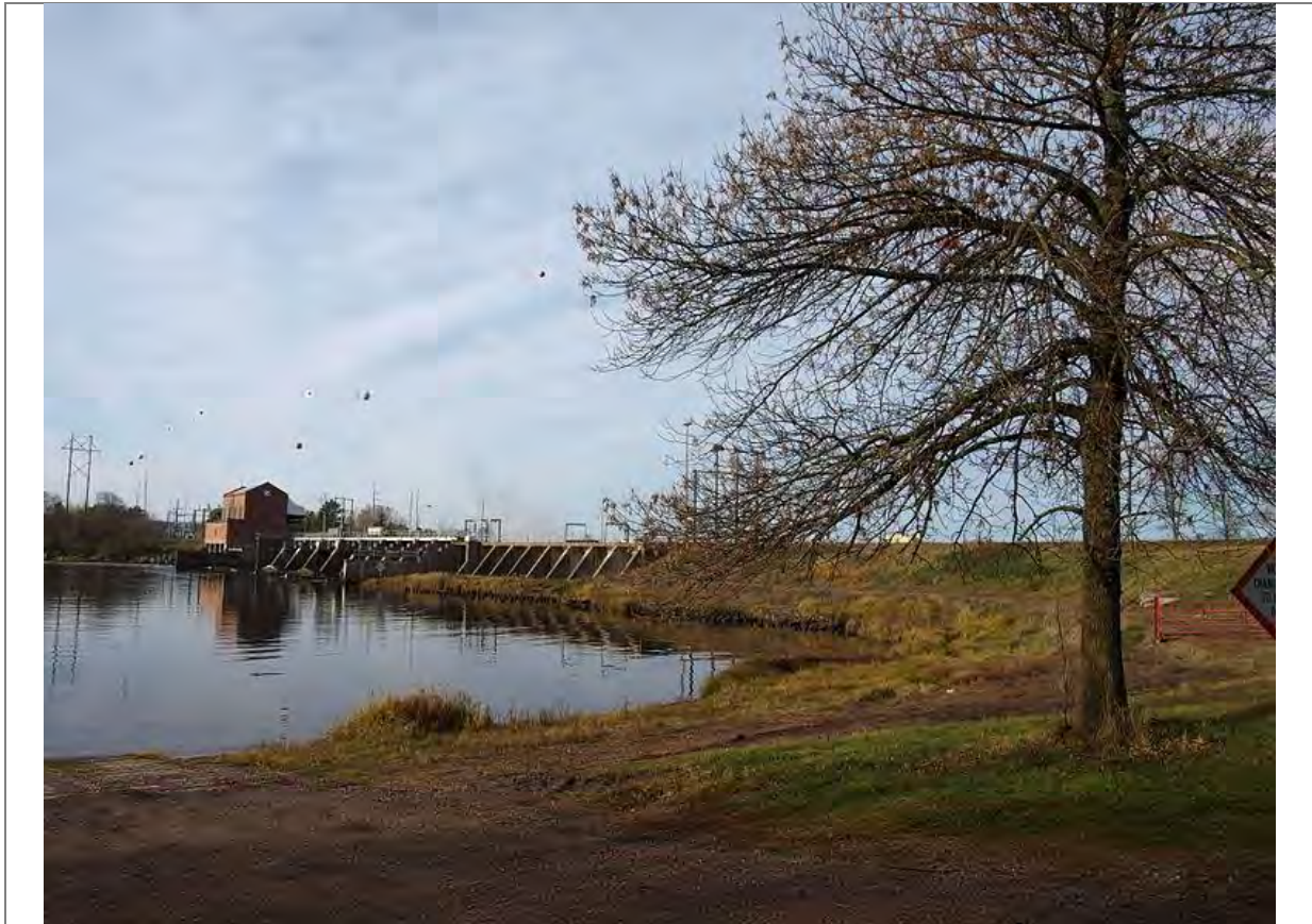
Photograph 3.1-1. Tomahawk Dam, viewed from downstream. Photo credit: Wikipedia
