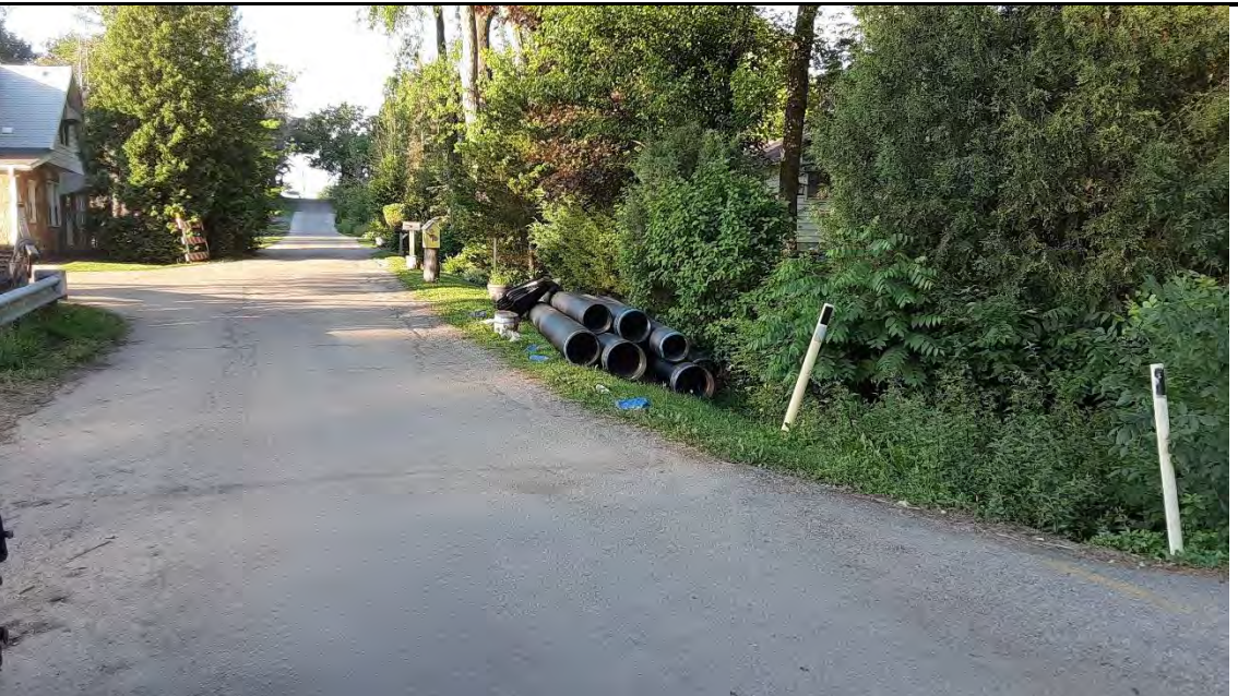
Replacement pipe and end sections along Poplar Drive
