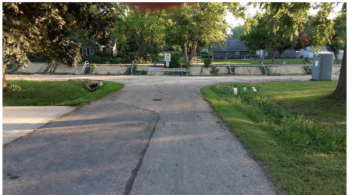
Stormwater inlet/ditch check SESC controls in place at Mulberry
