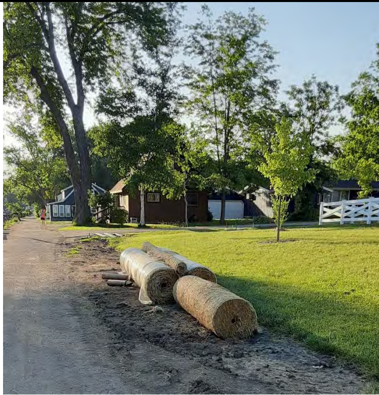
Temporary Erosion control blanket
