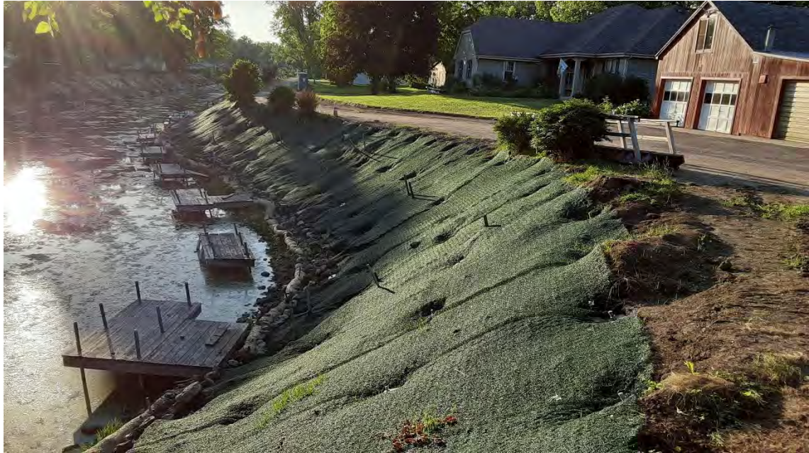
Close up of reinforced mesh and soil nails
