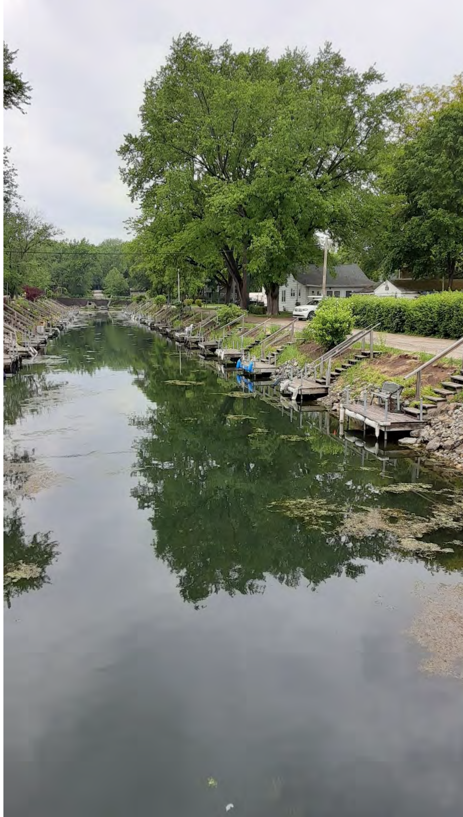
North embankment – North Channel Drive with no perimeter controls
