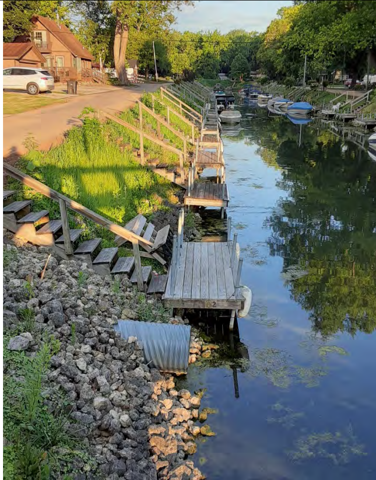
Cover vegetation in place, section stabilized
