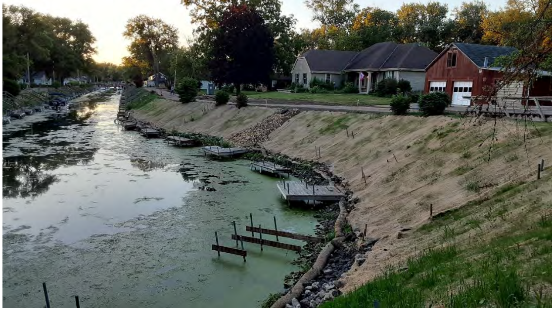
Closeup of a reinforced section, covered for vegetation establishment
