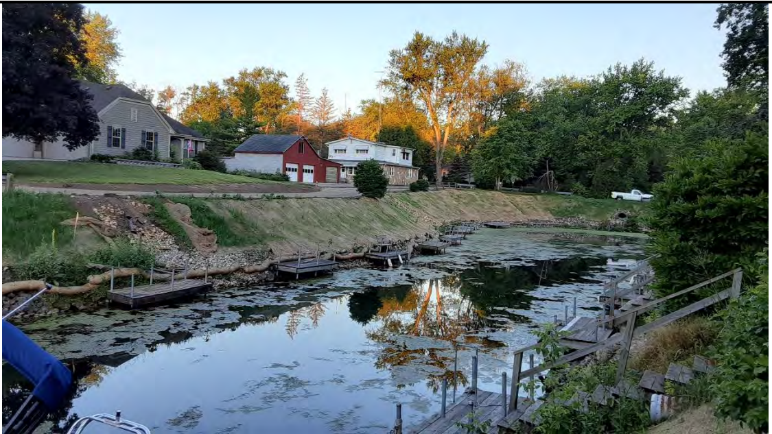
Blanket and cover over reinforced mesh area. Cover vegetation beginning to establish
