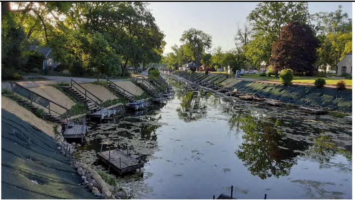
Inlet channel view east
