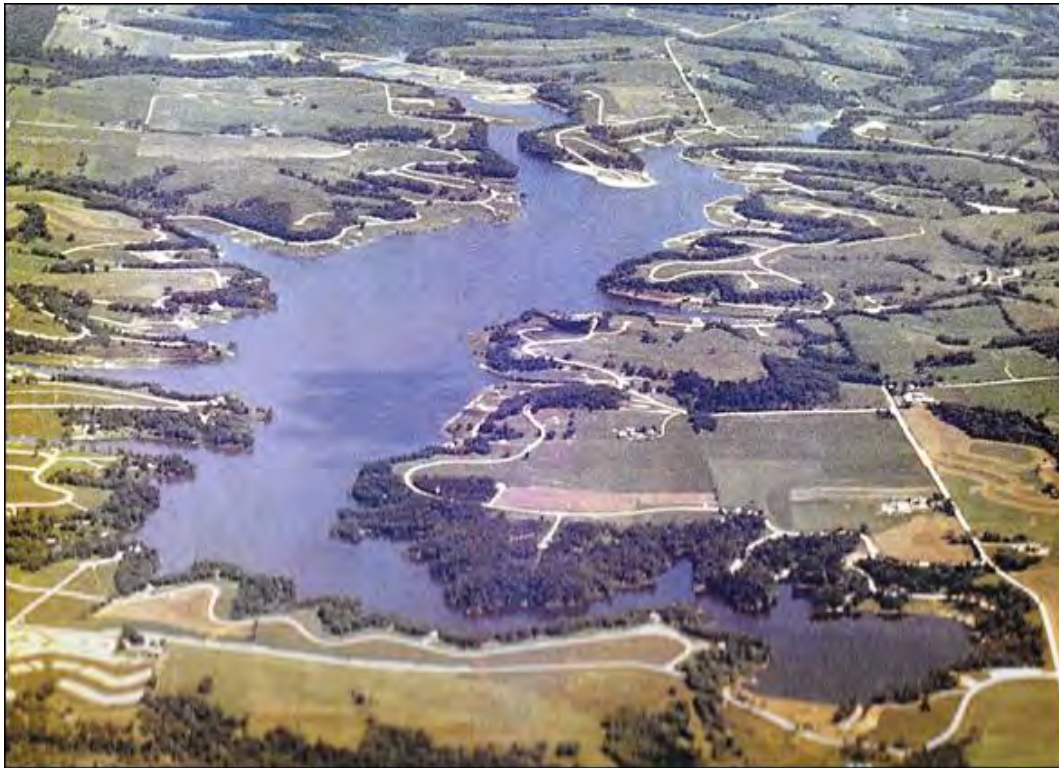
Figure 1: Lake Redstone shortly after filling. The two branches of Big Creek that flow into the lake are at the top of the picture. The dam is located at the lower right of the picture.
