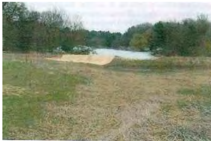
Figure 16- Sediment Trap at Mourning Dove Bay (Montgomery Associates Resource Solutions, LLC, 2011)
