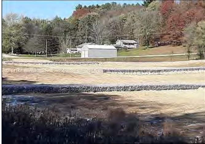
Figure 38: Stone-filled gabion baskets placed at the head of Mourning Dove Bay (LRPD Website)
