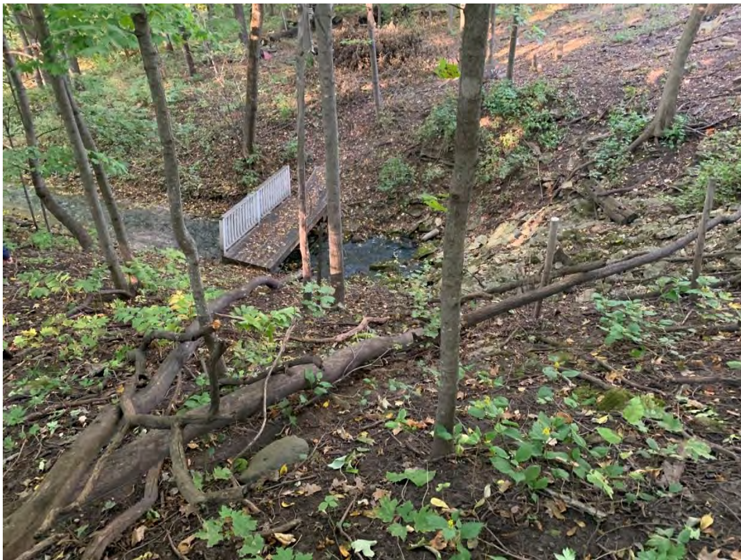
Photo 4. Cold-water spring originating at the base of a rock feature. Bridge will be removed.
