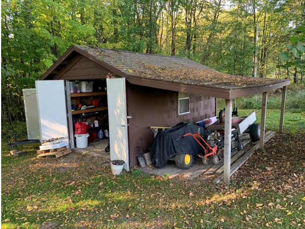
Photo 3. Utility shed/outbuilding – to be removed
