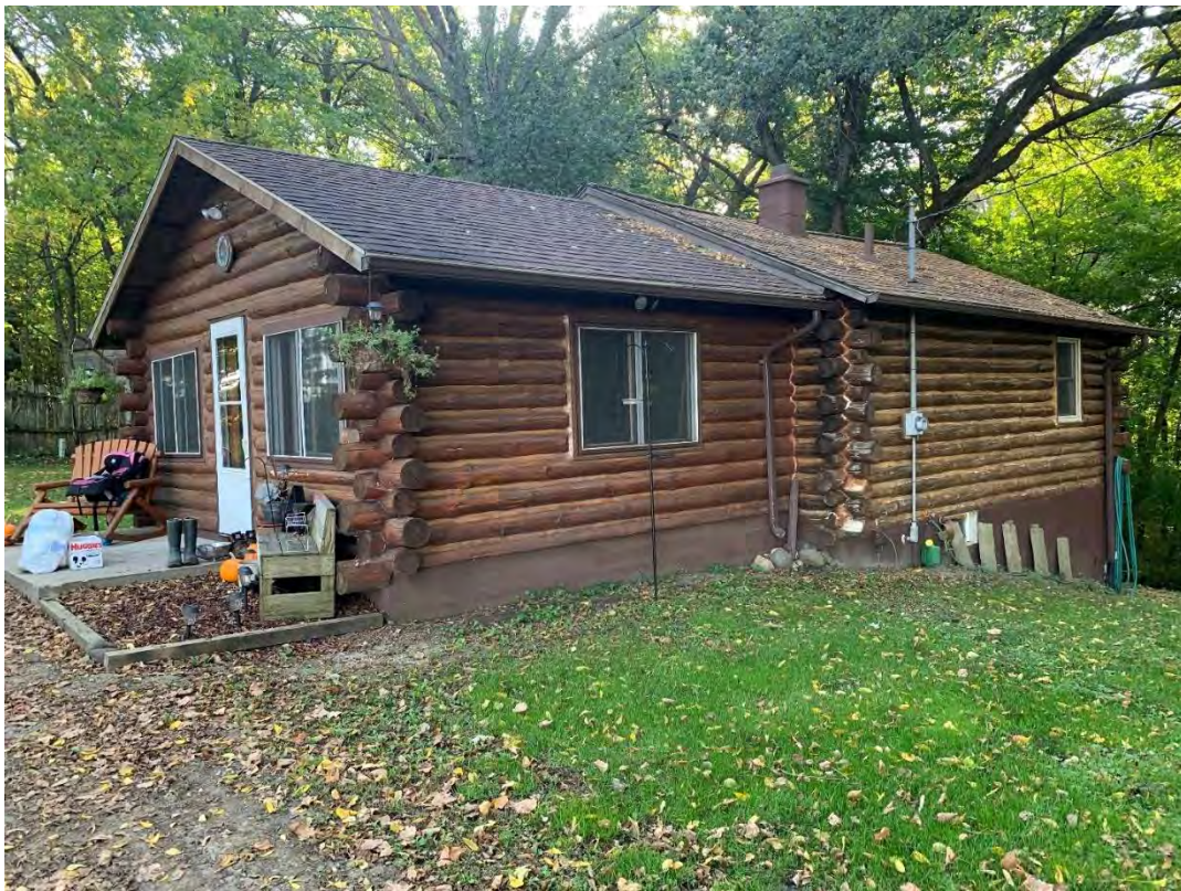
Photo 2. Residential home – to be removed
