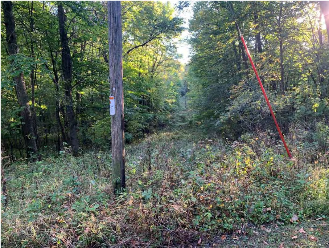
Photo 11. Distribution line bisecting wooded community
