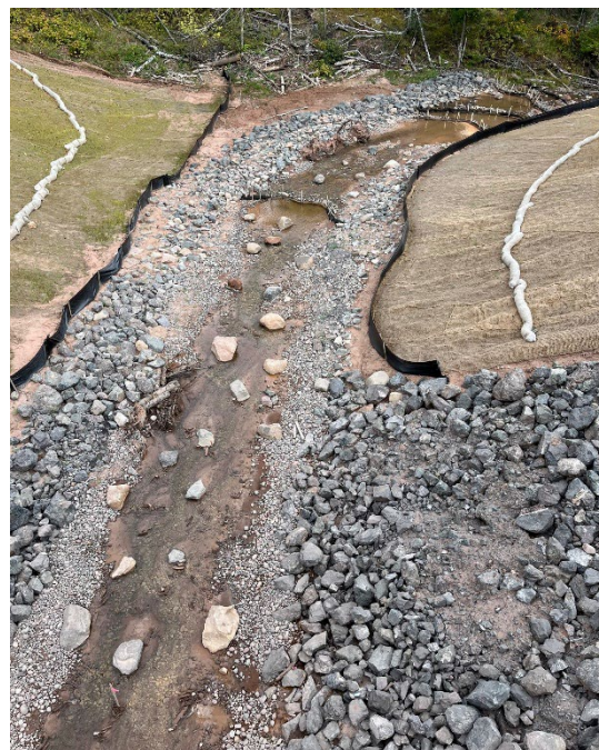
Construction at the Gandy Dancer State Trail was completed in fall 2024 to replace the deteriorating 315-foot-long concrete box culvert structure with a trail bridge over Little Balsam Creek. With this final barrier removed, 5.07 miles of class 1 trout waters are now reconnected, allowing fish to travel from Lake Superior throughout the upper reaches of the creek. Photo credits: DNR.
