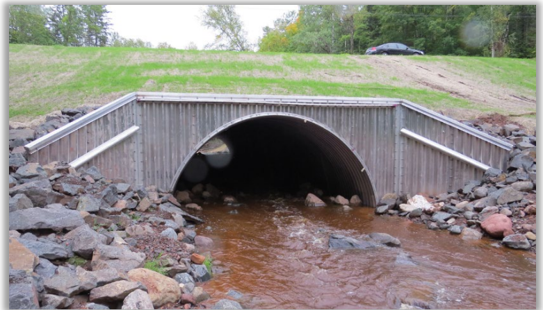
Replacement culvert for improved fish passage and flood water conveyance at Little Balsam Creek. Photo credit: DNR.
