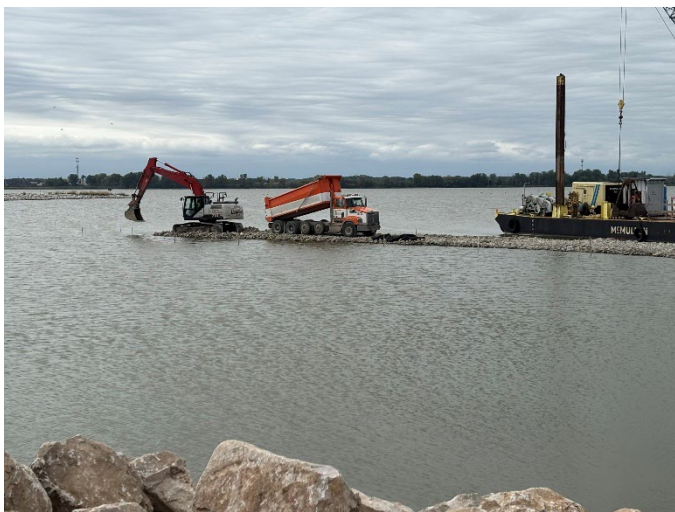
Construction on Cat Island in Green Bay. Photo credit: Brian Schuh, Ducks Unlimited (above and right).
