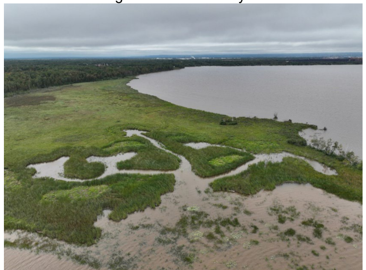
Restored hemi-marsh in Allouez Bay one year after construction. Photo credit: GEI Consultants.
