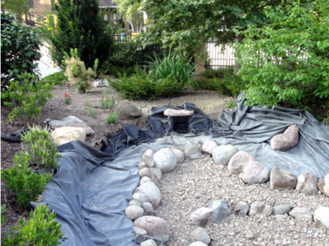
5. Inserting the skimmer to the pond for drainage of excess water.
