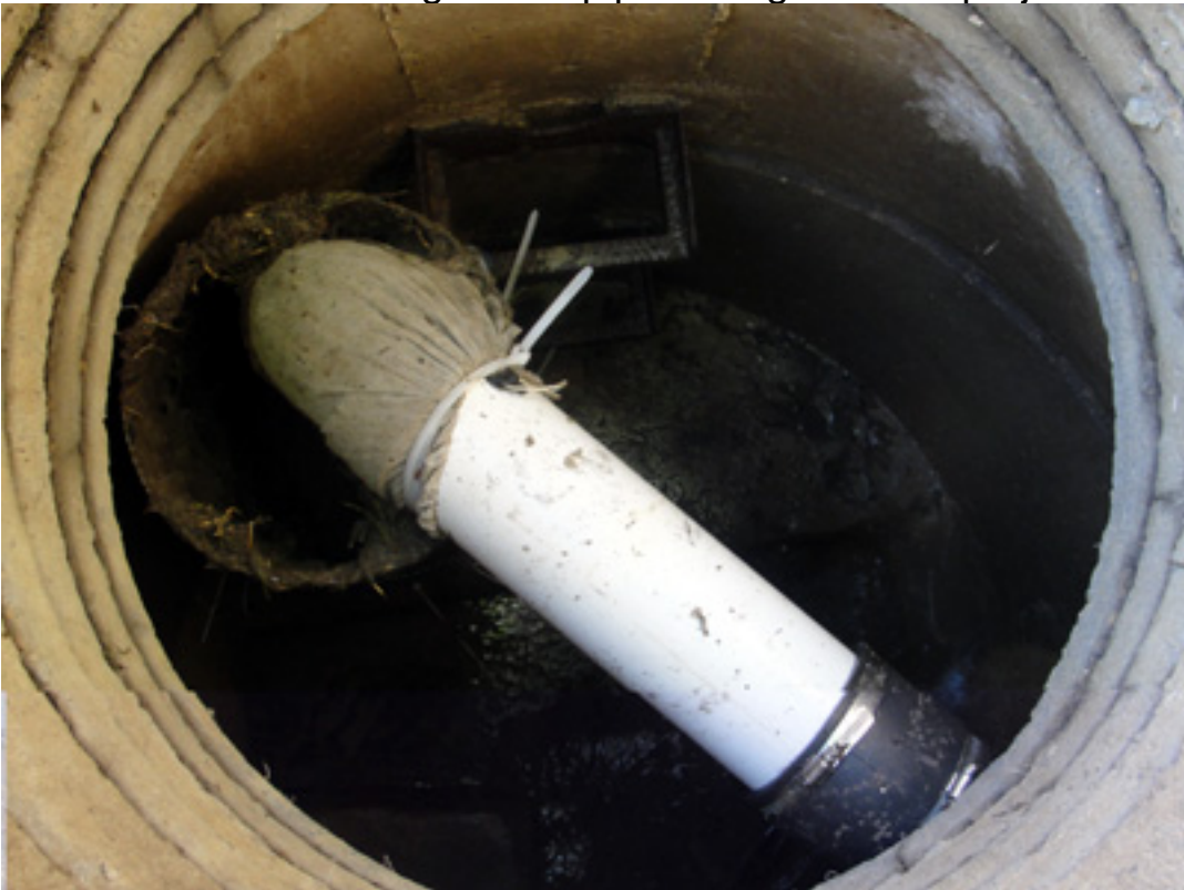
2.UW Physical Plant staff installed and ensured that the pond outlet has the secure filter bag on the pipe through out the project.
