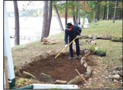
Photo 17. Installation of a small rain garden – Pine Lake.
