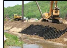
**Photo 10. Geoweb installation on streambank – SW Wisconsin.**
