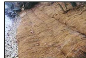
**Photo 11. Encapsulated soil lift installed on shoreline.**
