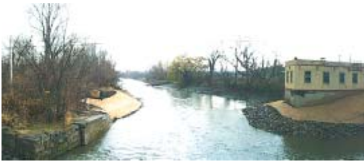
Baraboo River after removal of the Linen Mill Dam, courtesy of Konstantine E. Margovsky
