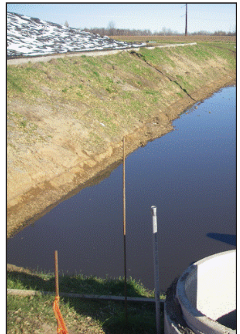
Silage Leachate Sediment Basin in the Mead Lake Watershed Photo Courtesy of WDNR
